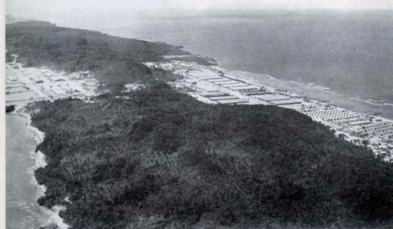
Fig. 11. The Naval Supply Depot (NSD), left, and the Advance Base Construction Depot (ABCD), right, on Calicoan Island.
