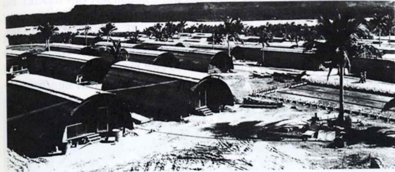
Fig. 5. The most common military structures built in Guiuan were the Quonset huts.
