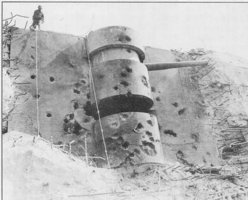
Effect of cruiser gun fire on casemate. Japanese fired rifles from these holes upon assault party until silenced by automatic fire from LSM. Note escape ropes.
