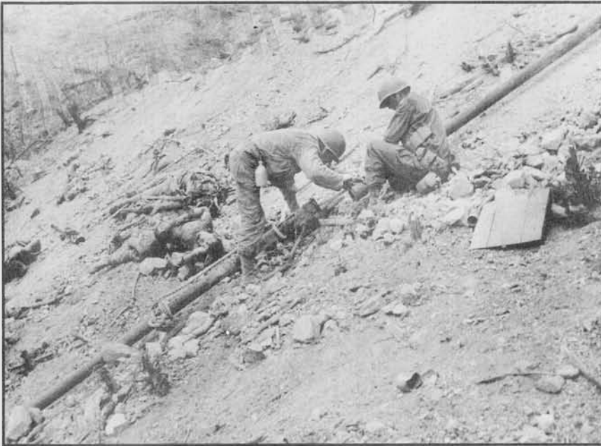
Fastening pipe together to pump oil into the mortar pits on CABALLO Island.
