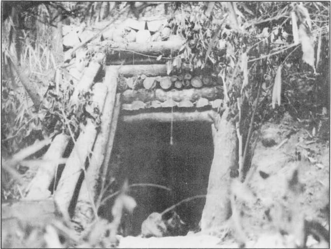
A reinforced dugout encountered by the 149th Infantry in the PILAR-BAGAC area.
