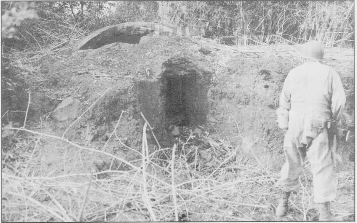
Reinforced pillbox destroyed by 151st Infantry vicinity PARANG
