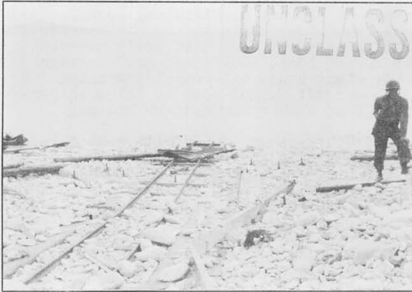
Minefield on beach at Corregidor lifted by Company B 113th Engineer (C) Battalion during mopping up on the Rock. Note Q boat launching tracks.
