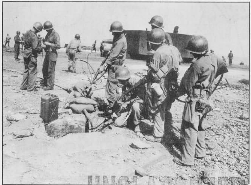
Placing hose nozzle and connecting demolitions.
